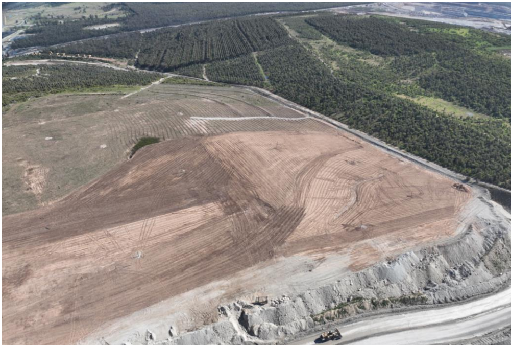
Figure 4 Northern Rehab Area after topsoil and stag trees
